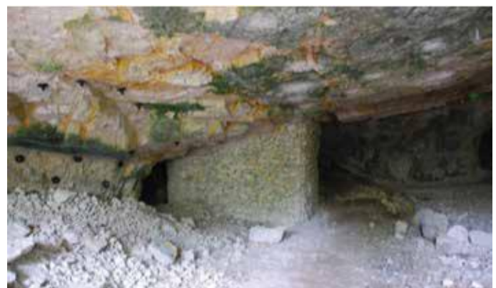
Fig. 4. Finished pillar, source: own elaboration
